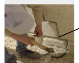
If you don't want the electrical wires to show, you can place them in the joints between the stones before putting in the mortar.
