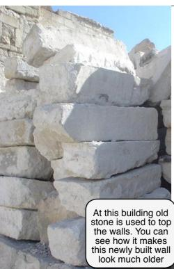
• Used very old and weathered looking stone to cap the exterior stone walls (building walls as well as exterior garden walls). This will help the newly built wall blend in better with the old walls.
