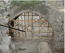
• It is important to check what kind of cracks you are dealing with. Some are very old cracks and are not dangerous. But other newer cracks may be dangerous. • Small cracks can be filled in with a mixture of a proper lime mortar and powder that is made from the original rock. This mixture looks like the stone that it is filling in.
